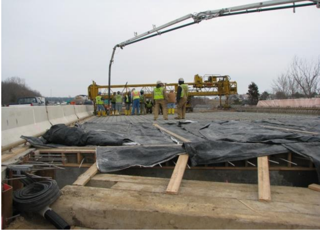
Figure 11 Curing blankets for concrete curing.
