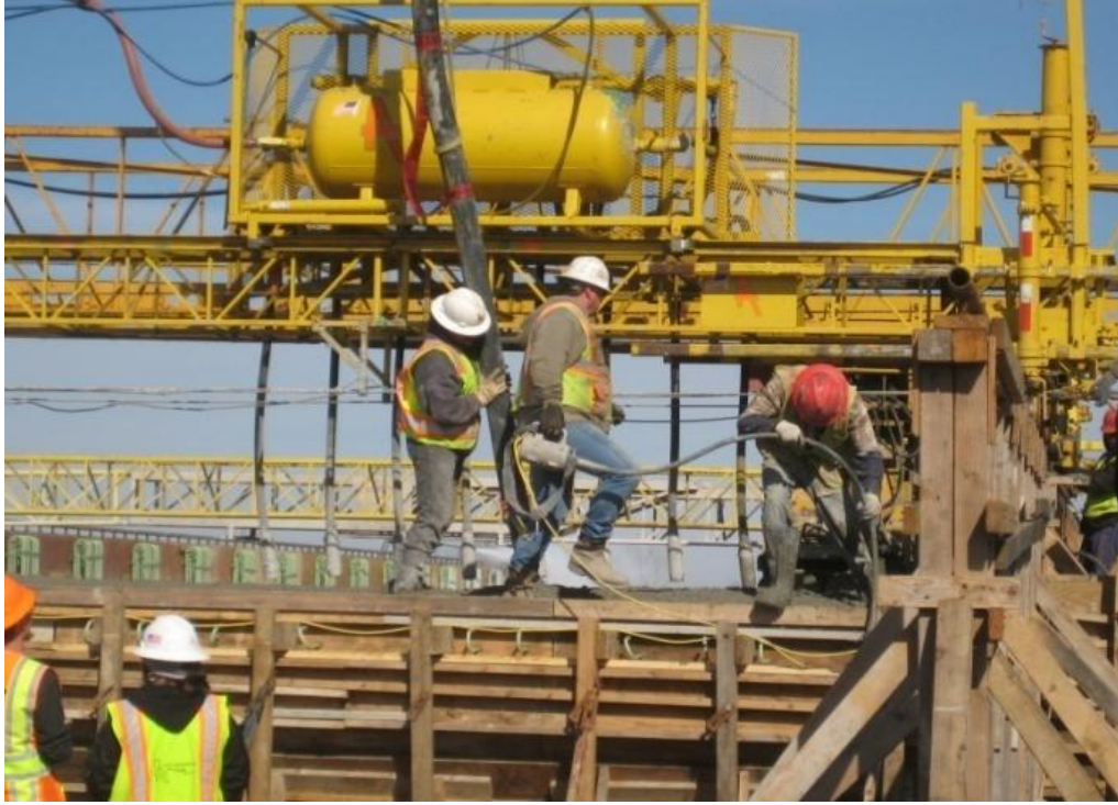
Figure 7 Construction crew placing concrete pouring and vibrating.
