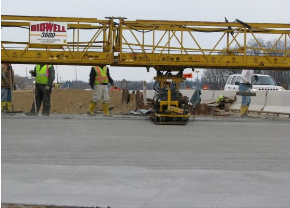
Figure 9 Concrete being finished.
