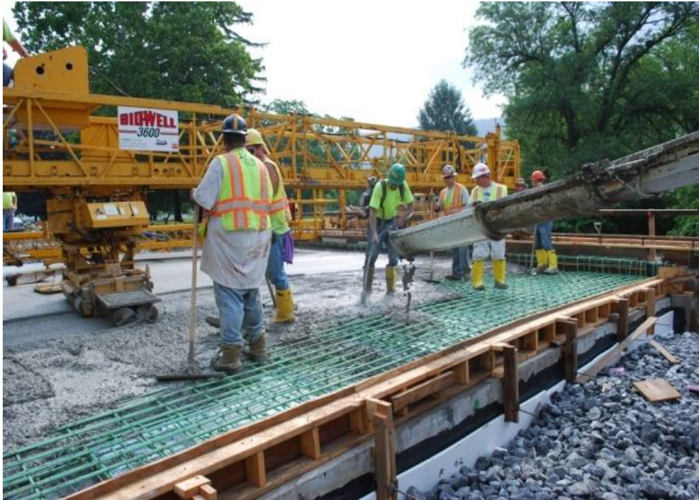
Figure 12 Concrete being vibrated.
