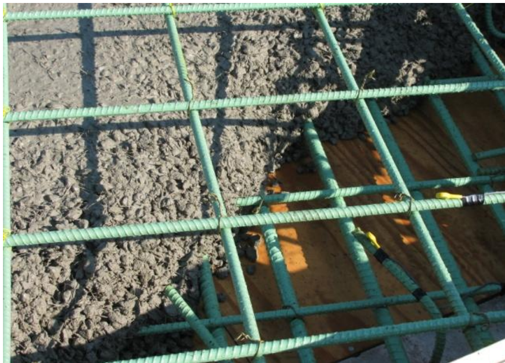
Figure 10 Two i-buttons being placed.
