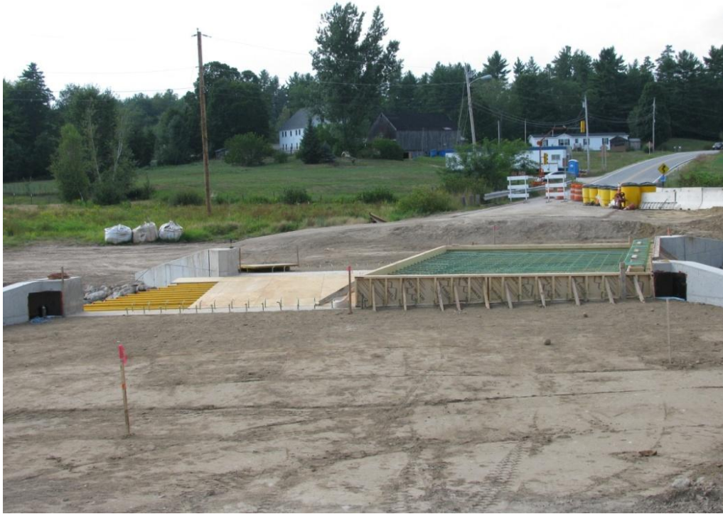
Figure 1 Route 107 bridge deck in Epsom, NH.
