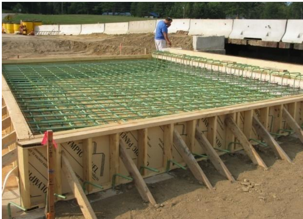
Figure 6 Bridge deck with removable wood form.
