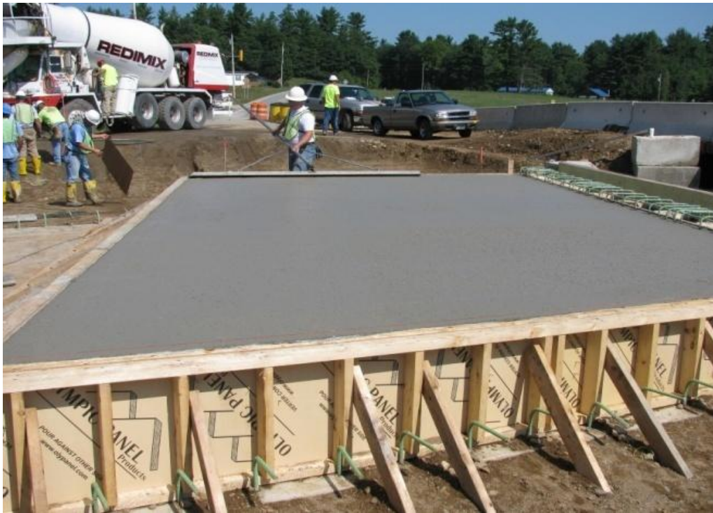
Figure 12 Concrete being finished.
