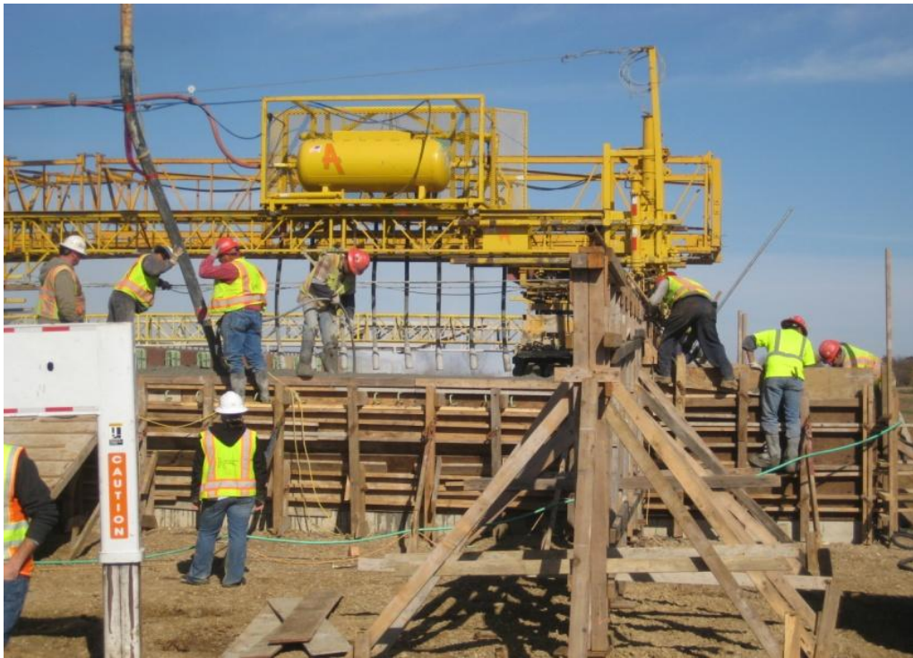
Figure 10 Concrete being placed and vibrated.
