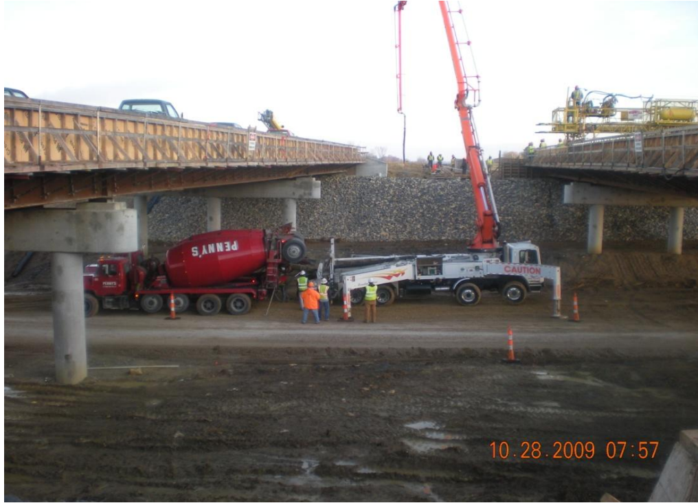
Figure 1 US-59 Bridges (Southbound-left and Northbound-right).
