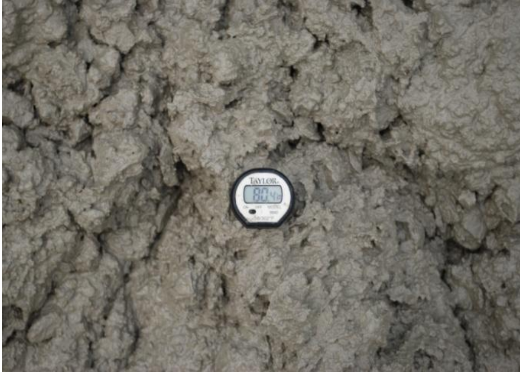
Figure 13 Concrete temperature being tested by sensor.
