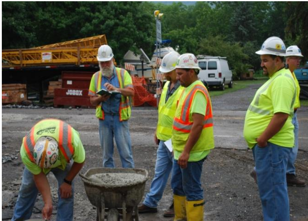
Figure 6 Concrete being tested by Penn DOT technicians .
