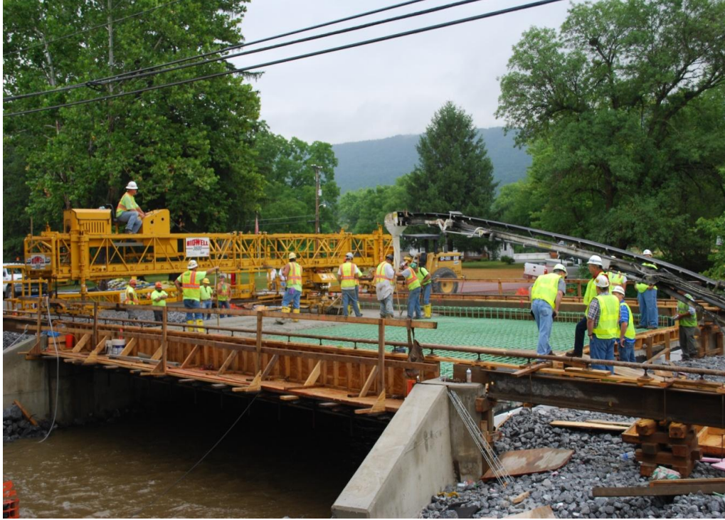
Figure 1 State Route 36 Section 20 bridge deck.
