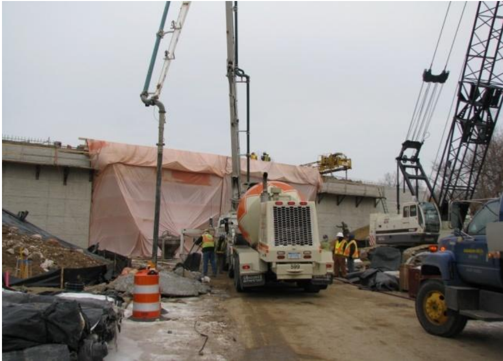
Figure 10 Concrete heated tent enclosure.
