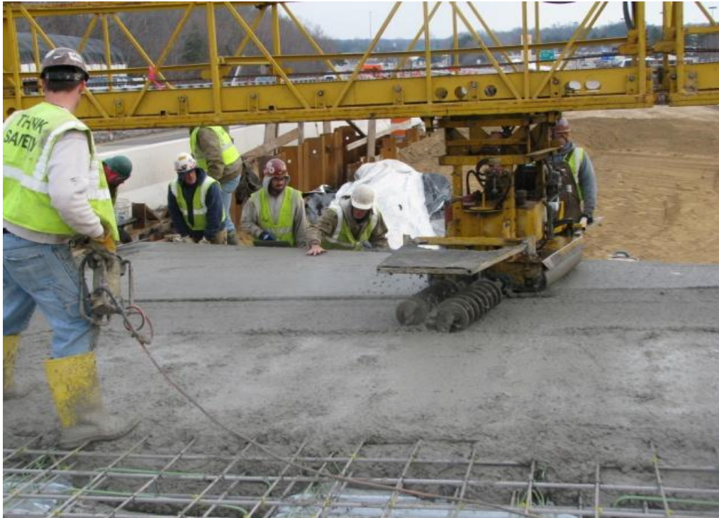
Figure 8 Concrete being placed.
