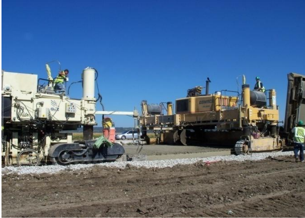
Figure 9 Concrete passing through the paver.
