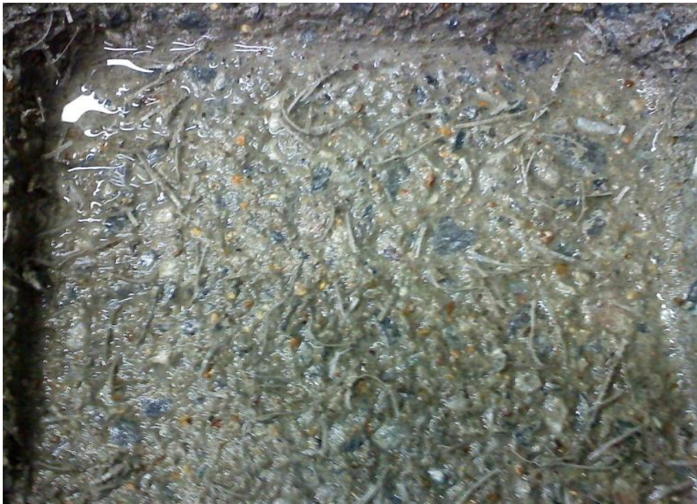
Figure 21 NH salt scaling sample after 50 th freeze-thaw cycle.
