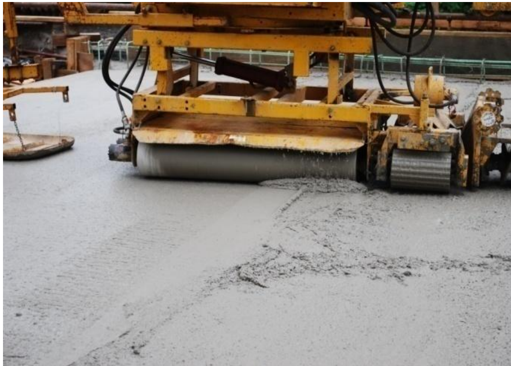
Figure 10 Concrete being finished.
