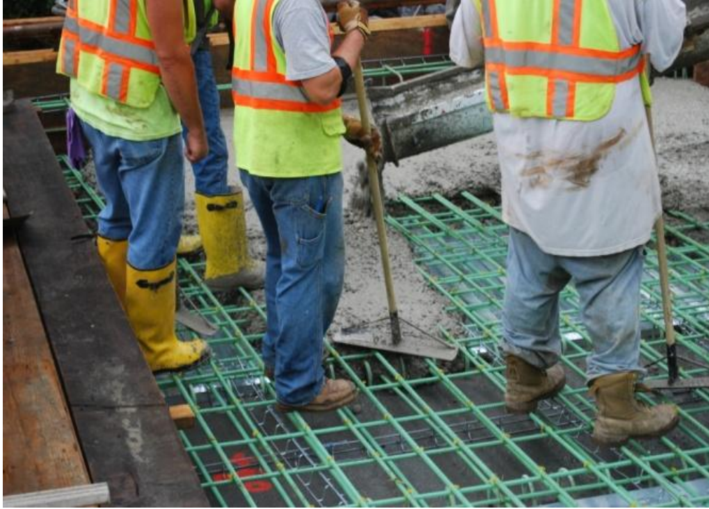
Figure 7 Concrete being spread by construction crews.
