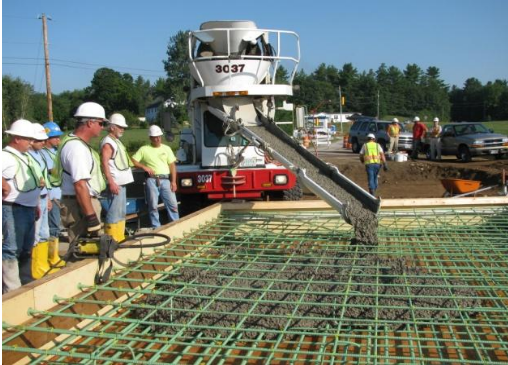
Figure 7 Concrete being placed.
