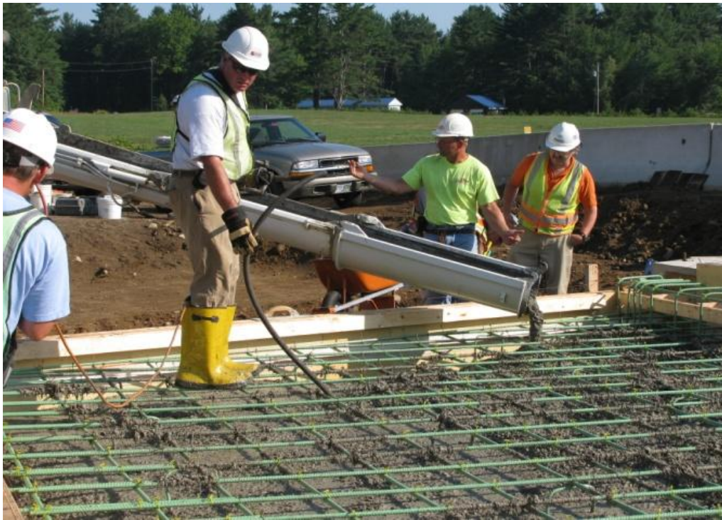
Figure 8 Concrete being vibrated.
